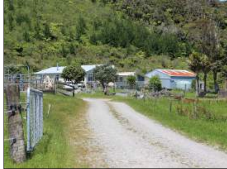
2.0: Existing farmhouse and ancillary buildings on site.
